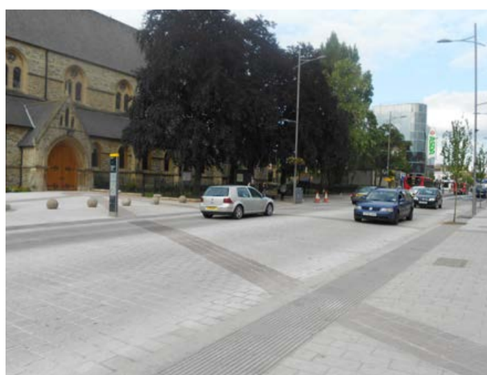
Flat top table - Flush flat top speed tables linking lateral public spaces at key nodes and gateways
